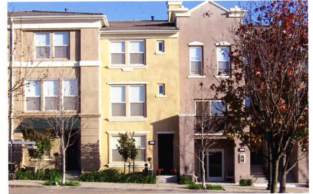
Variety of rooflines
