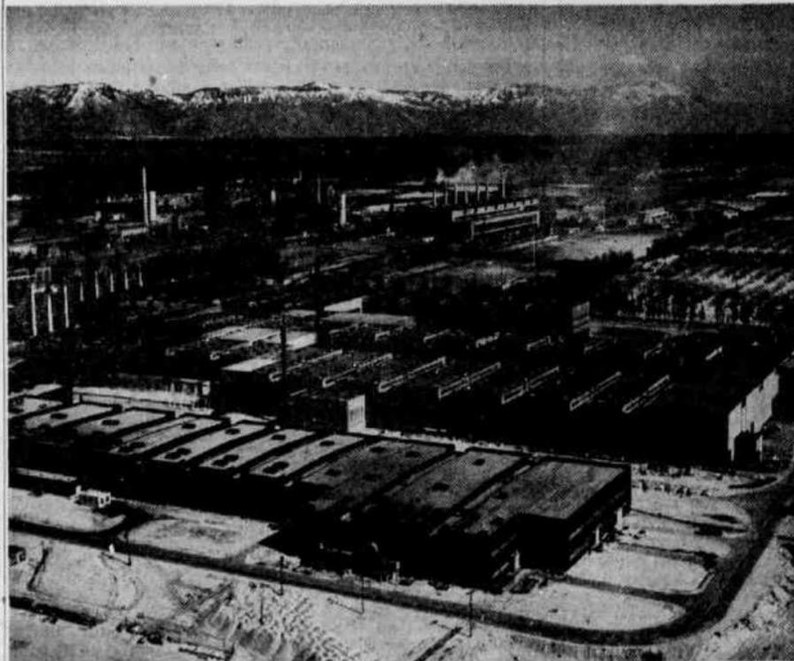
PANORAMA OF KAISER PLANT—Here is an aerial view showing a part of the vast Kaiser steel empire at Fontana. Plate, strip and pipe mills are in the foreground. Upper left are the coke ovens and blast furnace while the open hearth stacks, seven of them, shown in the center. (Pacifio Air photo)
