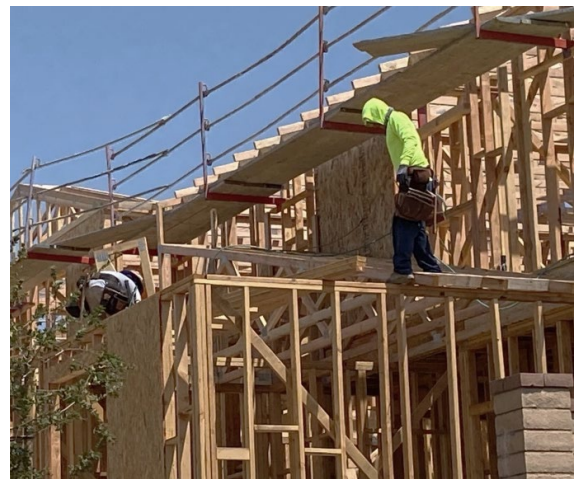
Construction workers building housing
