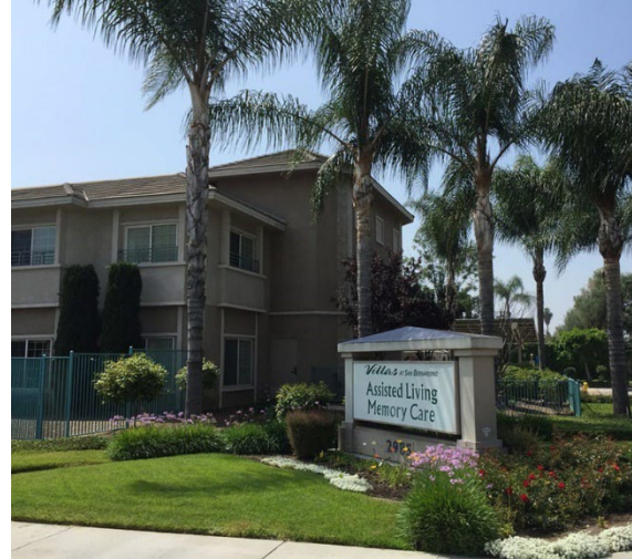
Assisted Living Facility in San Bernardino
