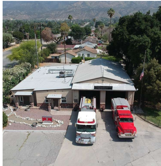
Del Rosa Fire Station
