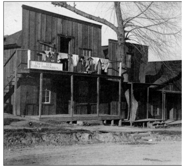
Photograph of original San Bernardino Chinatown
