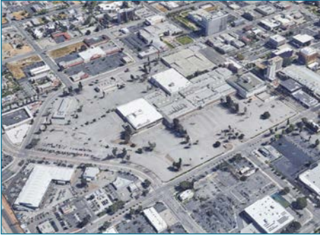
Carousel Mall Development Site
