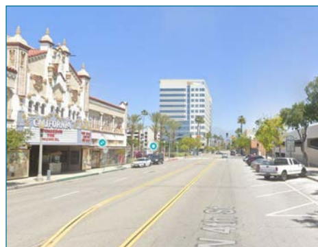
Existing Conditions Photo
