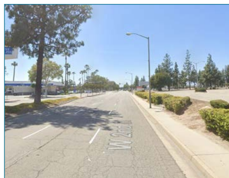
Existing Conditions Photo
