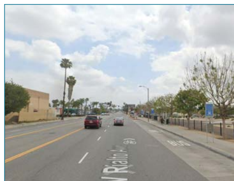
Existing Conditions Photo
