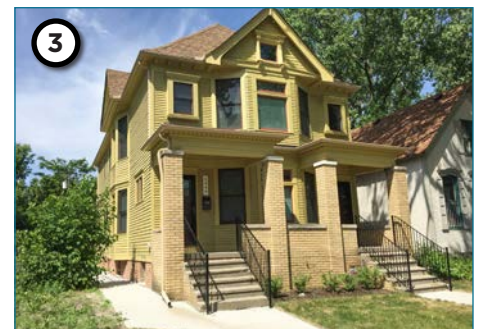
Cottage-style duplex home
