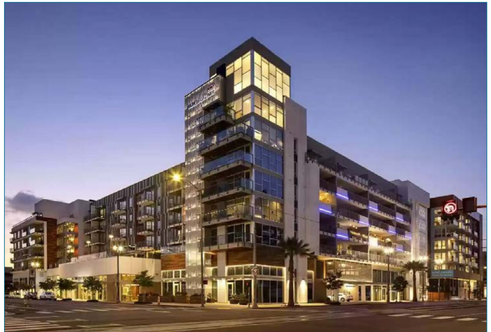
High-density mixed-use residential building with prominent corner treatment.
