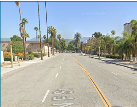
Existing Conditions Photo
